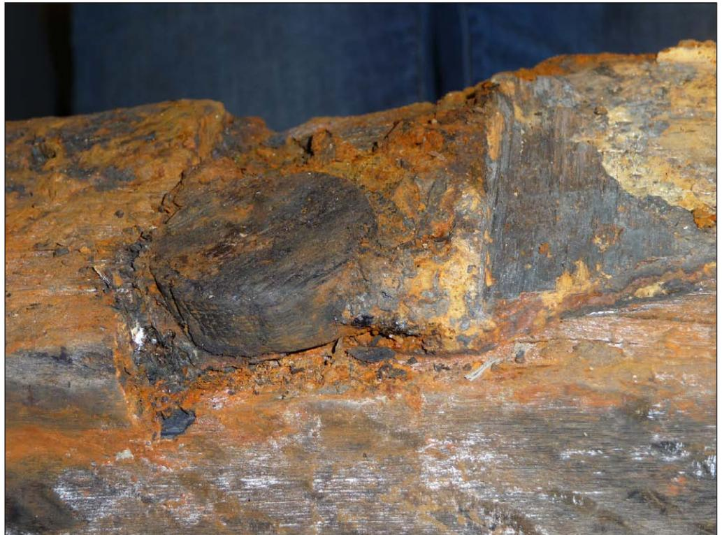
Filler plug located under frame FNFS 15-0 **B**
