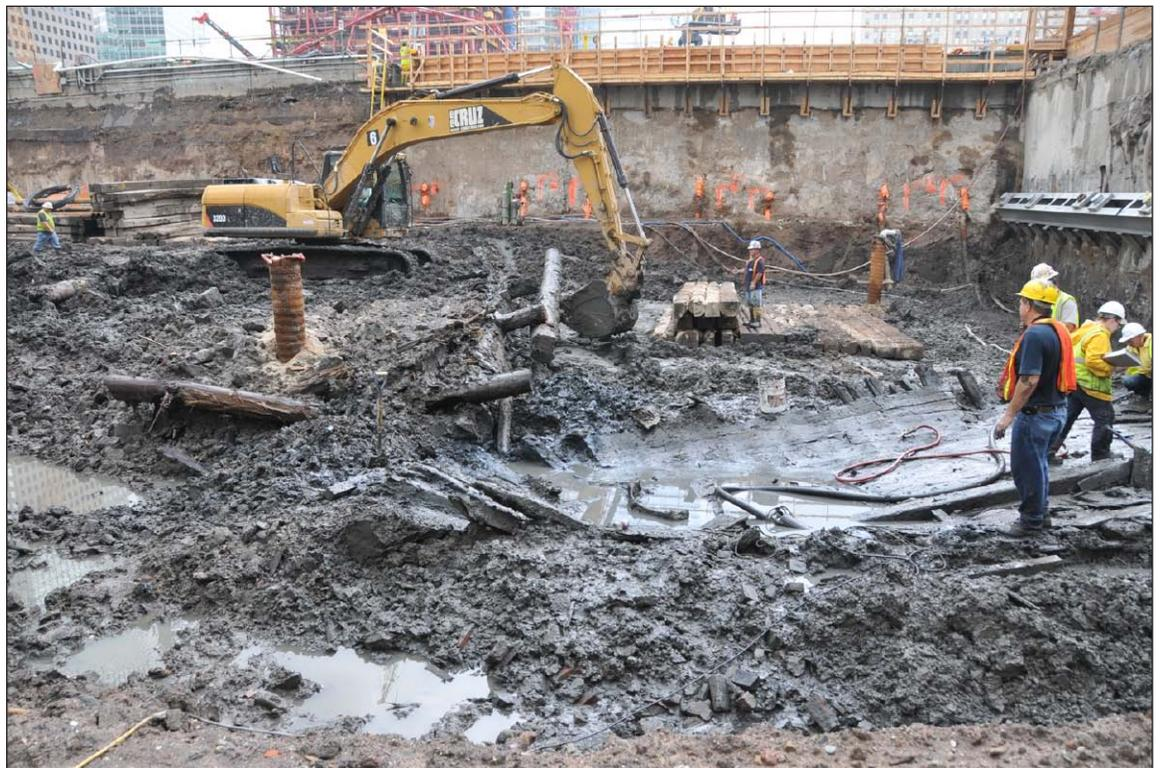
Facing north during removal of top course of landfill retaining structure north of ship remnant (in foreground). WTC slurry wall is in background and demising wall is to the right **B**
