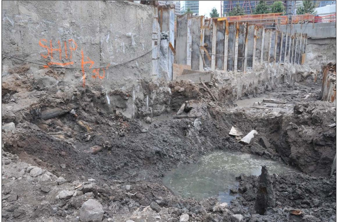
Block 54, to the east of the demising wall during excavation in the location where the remains of the bow were anticipated. The demising wall was marked to alert the backhoe operators to the possible presence of the bow.
